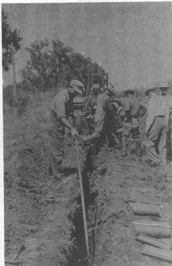
Laying Telephone cable in early 1900's
