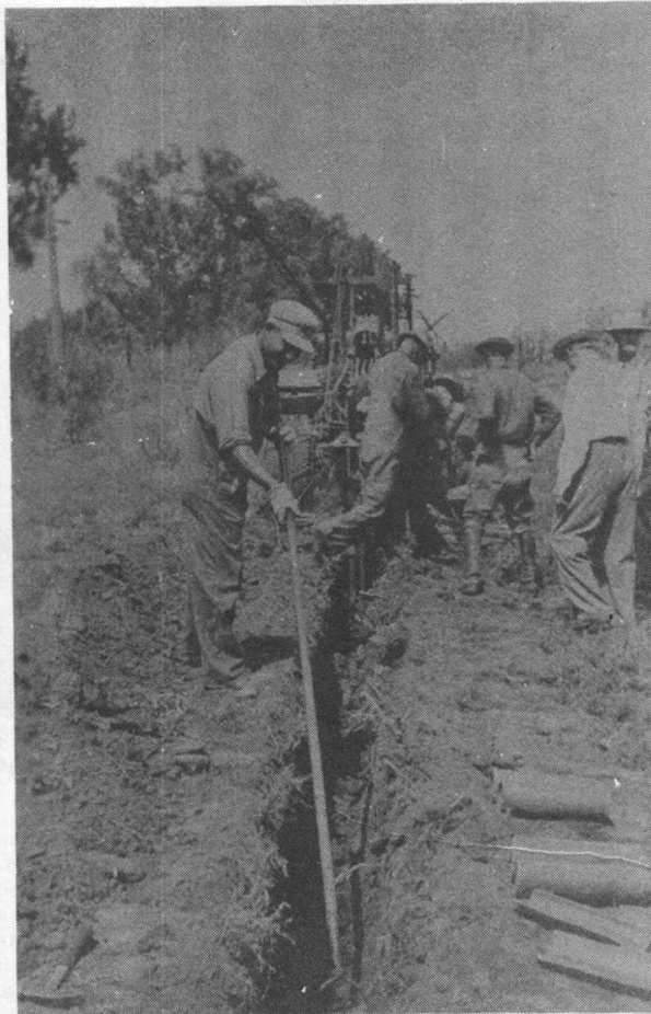
Laying Telephone cable in early 1900's
